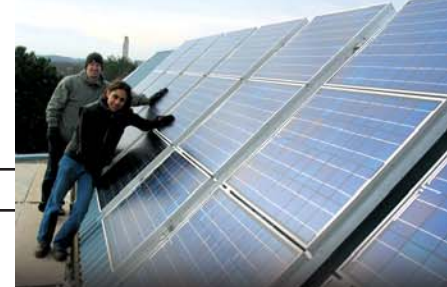
Students helped install the Federation Hall photovoltaic solar array.
